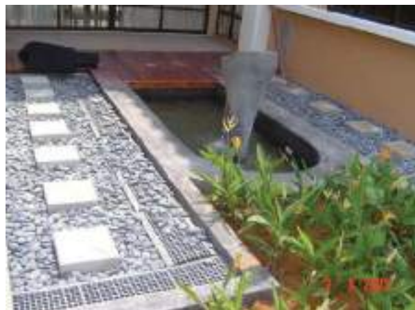
COMPLETED POND AT SHOW HOUSE
