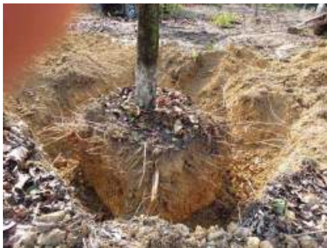
After do the trenching work
