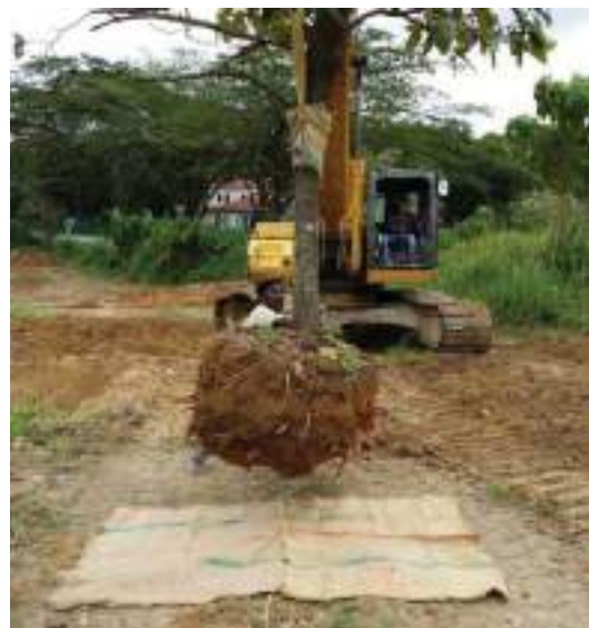
Used jute bags to wrap the root ball to protect tree roots
