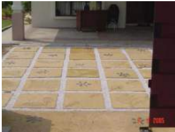
RC SLAB WITH LEAF IMPRINT AND PRECAST
